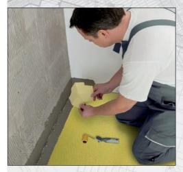
being laid, it is recommended that they be protected from loading by laying boards on them. Other protective measures may be necessary, too, e.g. protection from direct sunlight or rain in outdoor locations. Any water collecting in the texturing must be removed before applying thin-bed mortar.
