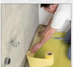
As soon as the DURABASE CI++ matting has been laid, tiles can be laid on top of it using a thin-bed technique and a thin-bed mortar appropriate to the flooring. Practically, it is advisable to apply mortar to the round depressions in one working step and then apply thin- bed mortar and roughen it in another. The work can also be done in such a way that the application of the top mortar layer only starts after the initial application has hardened.
